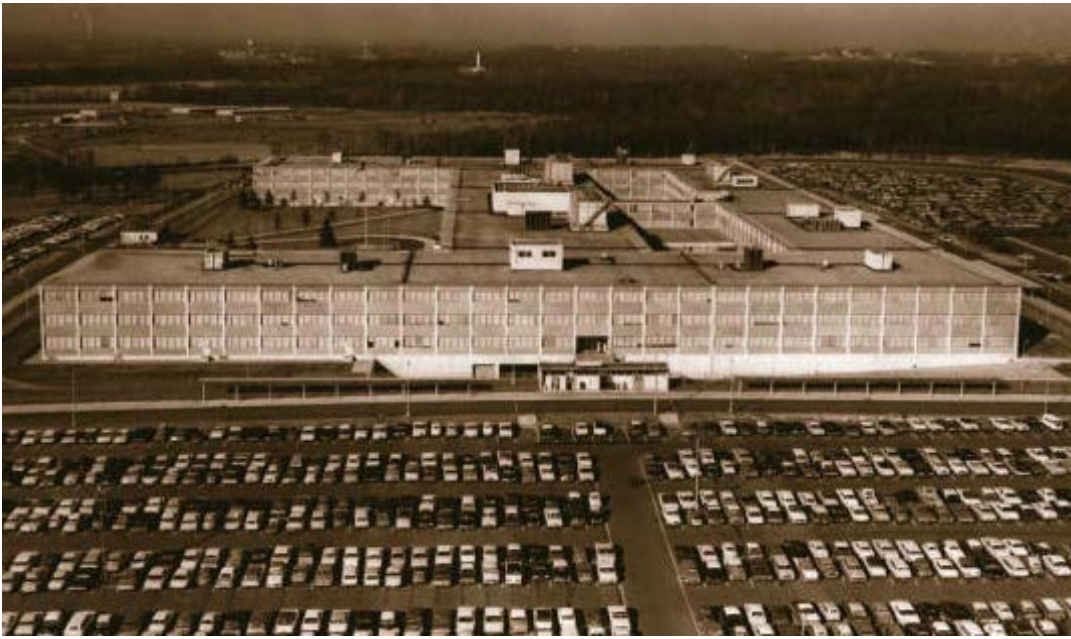
(NSA's Operations Building #1, Fort Meade, MD).
