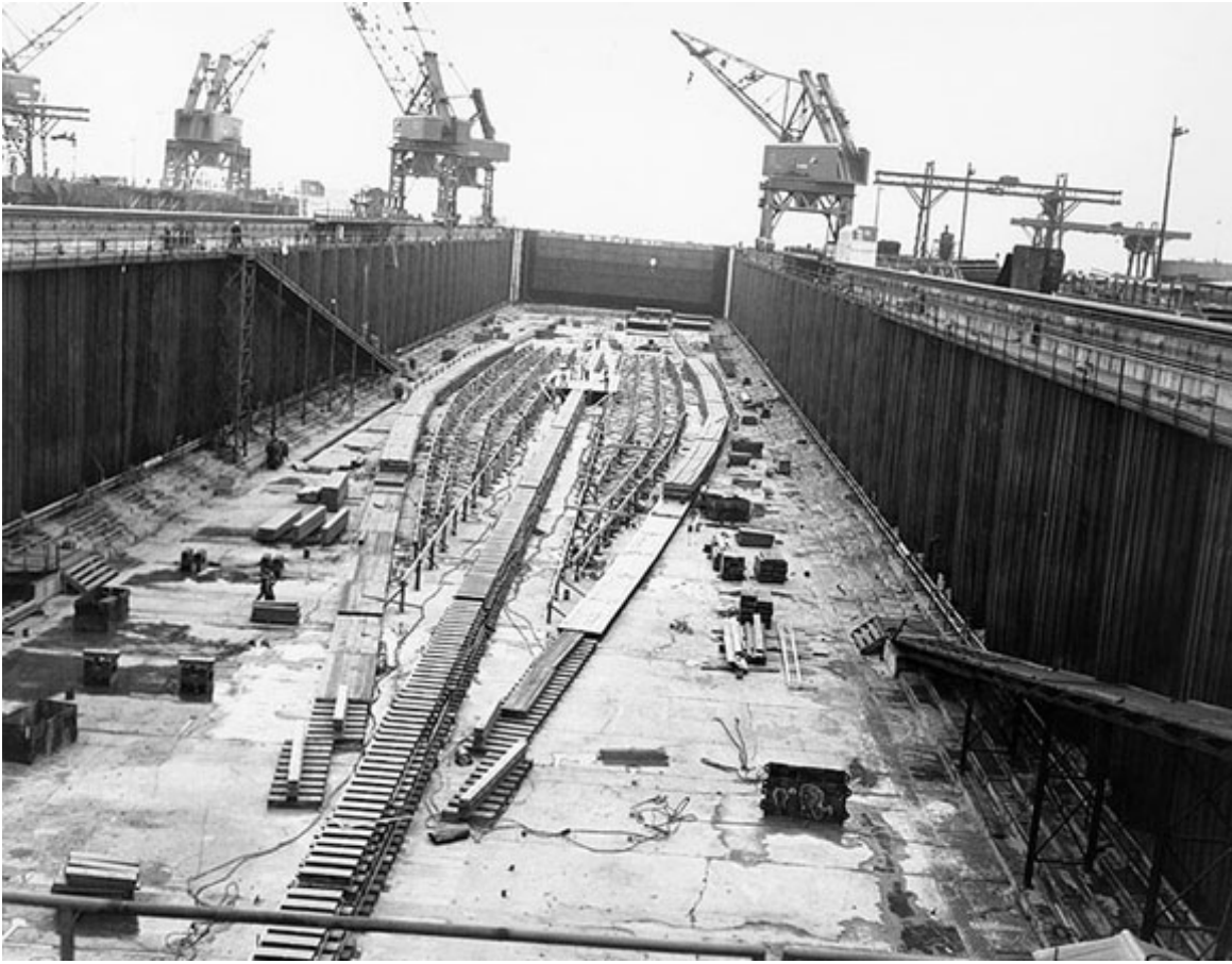
(USS United States , pictured in drydock with her keel laid. Official Navy Photo)
